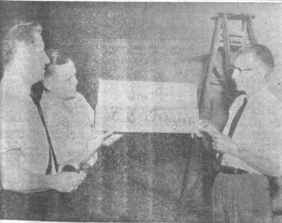
REMINDER OF THE PAST —Workmen remodeling the store formerly occupied by Vail and Baddour and 10 store found the signature of the late L. S. Traylor and the date 6/16-94 on a board in the walls. Mr. Traylor, father of the present L. S. Traylor of Iuka, worked for Capt. C. J. Hyatt who built the store building in 1868 and operated a mercantile business there until 1897. Capt. Hyatt was the grandfather of W. J. Pyle of Iuka. Shown examining the signature which was carved out of the wall are, left to right, W. J. Pyle, Stewart Vail of Vail and Baddour Stores, and L. S. Traylor. The board was presented to Mr. Traylor as a memento.
